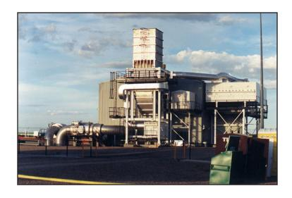
you lose efficiency," says Marie Standing, senior mechanical engineer with TransCanada. To remedy this, they installed an air-to-air heat exchanger on a turbine exhaust at the Compressor Station in Saskatchewan. The heat exchanger recovered heat from the turbine exhaust and used it to preheat a portion of the inlet air to 385°F. This in turn mixed with the remaining cold inlet air to bring the entire inlet airstream up to 75°F, allowing the turbine to gain hundreds of horsepower.
