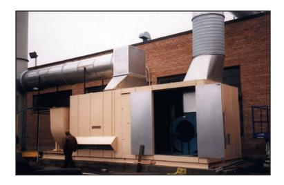
Each heat exchanger is actually part of a complete packaged heat recovery system that also includes supply and exhaust fans, dampers, and filters.
