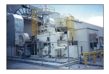
turned to Plymouth, Michigan-based Durr Environmental, a manufacturer of air pollution control systems that had previously supplied equipment for the facility. Des Champs supplied the VariMax™ system, an indirect-fired recirculating gas heater. A burner in the combustion chamber generates heat, and the combustion products recirculate by means of a fan, rather than flowing straight up a stack.
