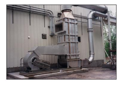
air comes from the process at 900°F – hot enough to burn the bags – and it must be cooled to 250°F. Previously, with the existing line, outside air was mixed with the hot air to cool it. A second line doing this would have resulted in exceeding the baghouse capacity.
