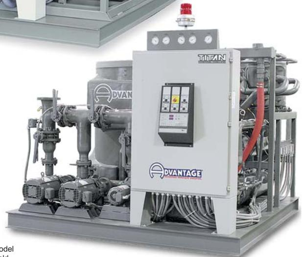
TI-60W shown. 60 ton water-cooled model with optional standby pump and manifold.
